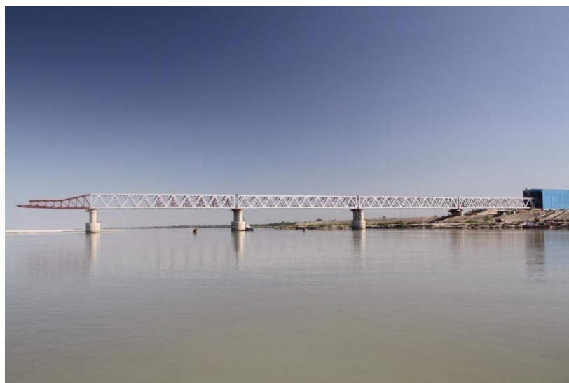
Launching of 4th girder span of Bogibeel Bridge
